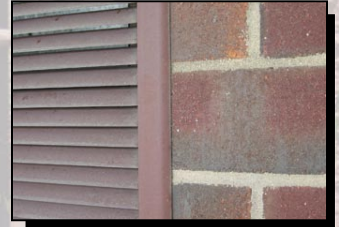
Two Inch Beveled Frame Tampers into Brick for Smooth Transition
