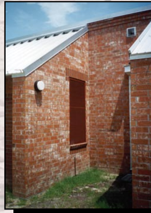
Brick Red Louver Recessed into School's Facade
